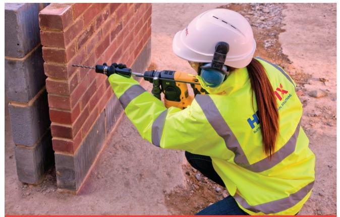
DryFix tie being power-driven into pilot hole
